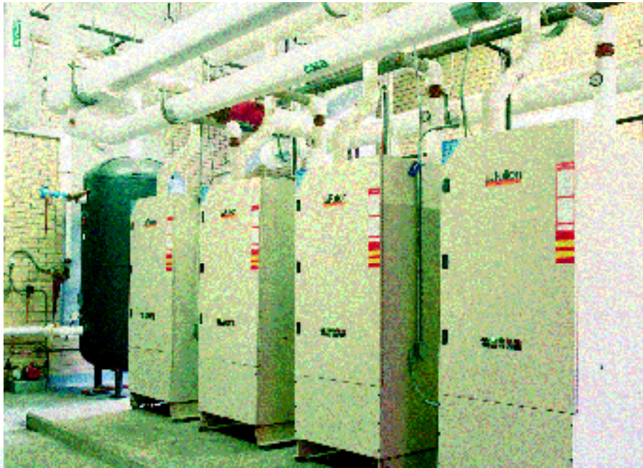
Modular installation of the four 1,000,000 BTU Fulton Pulse Combustion Boilers
